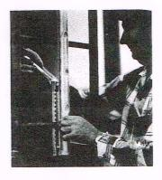
NOTE: AFTER FIRST SECTION OF CARRIER RAIL IS PROPERLY INSTALLED, THE INSTALLER MAY BUCKLE ON HIS SAFETY BELT, ATTACH HIMSELF TO A SAF-T-LOK SLEEVE, AND CLIMB UP TO INSTALL THE NEXT SECTION. BUT HE MUST EXERCISE EXTREME CAUTION TO SEE THAT HIS SAF-T-LOK SLEEVE DOES NOT RIDE UP OVER THE UNFINISHED END OF THE FIRST SECTION!
